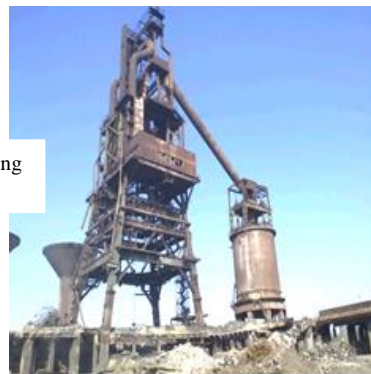
Fig. 2. Furnace assembly after preparation for blast
