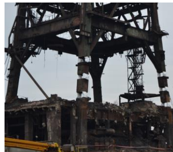
Fig. 4. Completing the preparation of metal pillars
