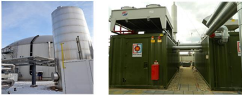
Fig. 3. (a) Digester for anaerobic degradation and. (b) Combined heat and power station (CHPS).
