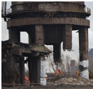
Fig. 5. Prepare concrete columns for supporting the purge bag
