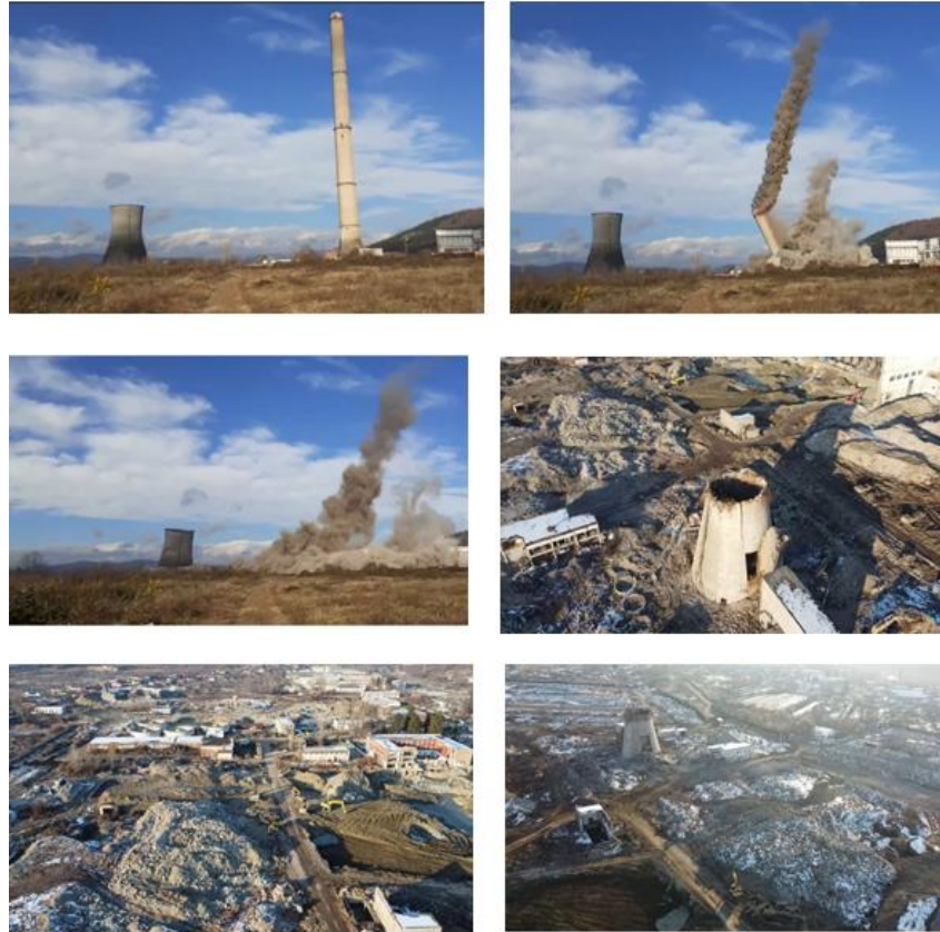
Fig. 3 The moments of the demolition of the Doicești-Dâmbovița Thermal Power Plant on caustobiolitic fossiliferous coal combustion (Source: editing - processing after A. Costea, 2022)
