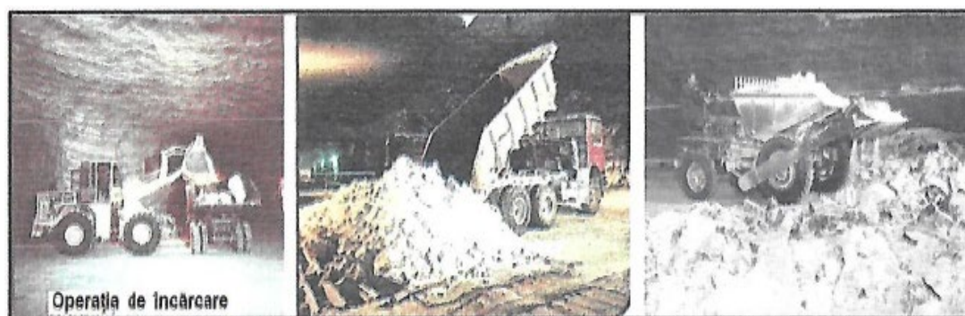
Fig. 14. Loading and transporting salt to the surface
