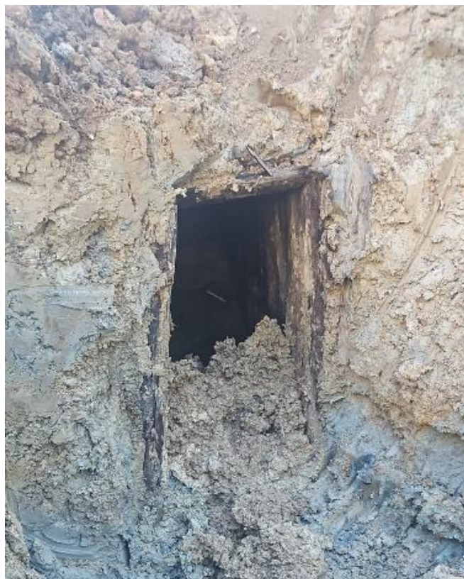
Fig. 3. Image of the drainage adit from Ferdinand mine
