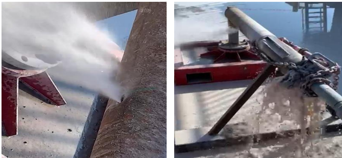
Fig.6. Perforation in the casing
