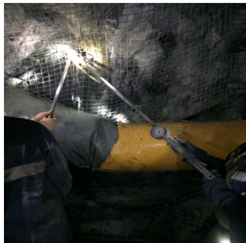
Figure 7. Applying of rock support to the 2 nd class
