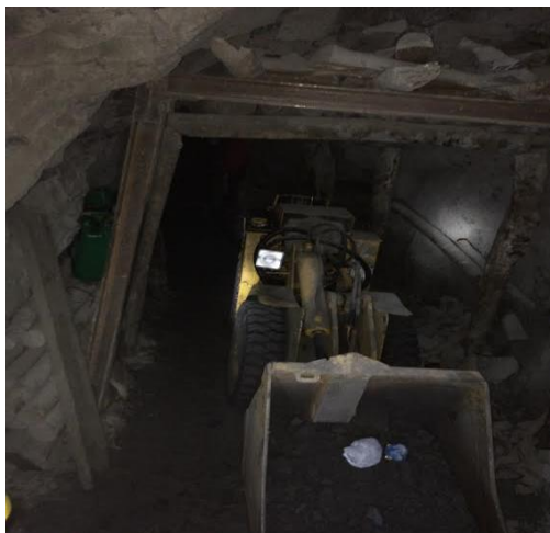
Figure 6. Applying of rock support to the 4 th class
