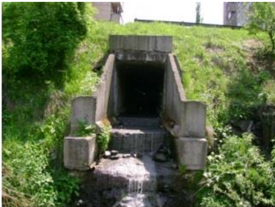
Figure 4. Discharge of domestic wastewater from a residential quarter in Lupeni directly to the emissary [1]
