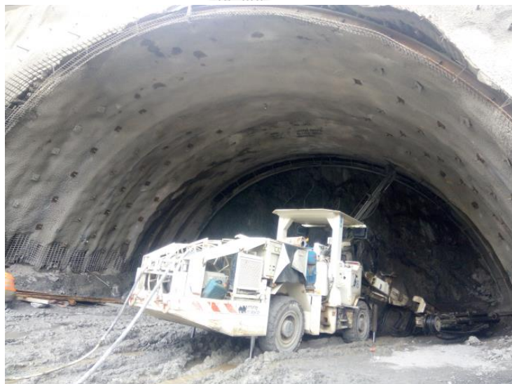
Figure 5. (b)- Phase 2: Making an excavation along the recommended circle on the upper half, Application of a wire mesh (150 * 150 * 6.5 mm). HEB 220 steel cladding, Surface coating with 35 cm shotcrete, Temporary Slab, wire mesh and shotcrete casting and IBO bolt application
