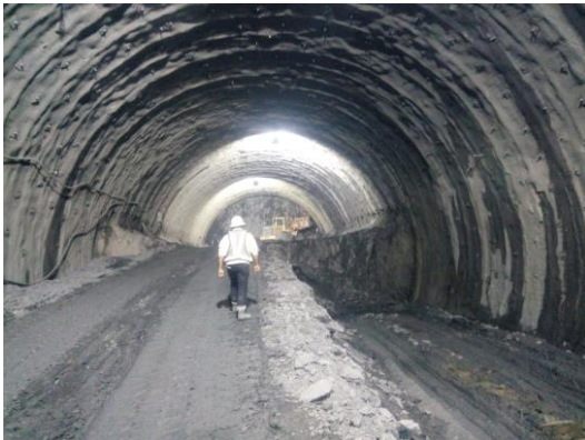
Figure 5. (c)- Phase 3: Excavation along the recommended circle on the lower right-lateral half, Application of wire mesh (150 * 150 * 6.5 mm). HEB 220 steel cladding, Surface coating with 35 cm shotcrete, and IBO bolt application
