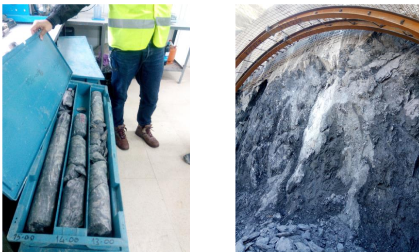
Figure 2. View of the decomposed new-low degree flysch units from the TBH-1 survey
