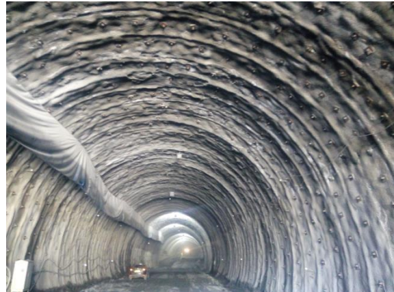
Figure 5. (e)- Phase 5: Execution of an excavation along the recommended circle on the base/ Slab, Application of a wire mesh (150 * 150 * 6.5 mm). HEB 220 steel cladding, Surface coating with 35 cm shotcrete, and IBO bolt application
