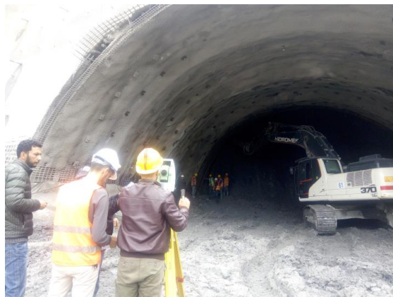
Figure 6. (c): Photograph of the Tachometer, e.g. "Leica, TS 09" of the tunnel underground monitoring
