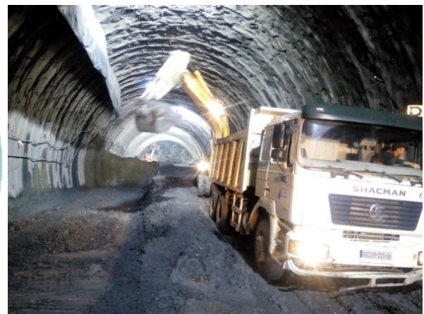
Figure 5. (d)- Phase 4: Making an excavation along the recommended circle on the lower left-lateral half, Application of a wire mesh (150 * 150 * 6.5 mm). HEB 220 steel cladding, Surface coating with 35 cm shotcrete, and IBO bolt application
