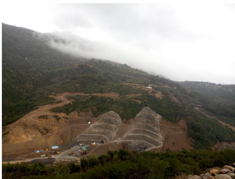
Figure 3. Photo of the tunnel portal
