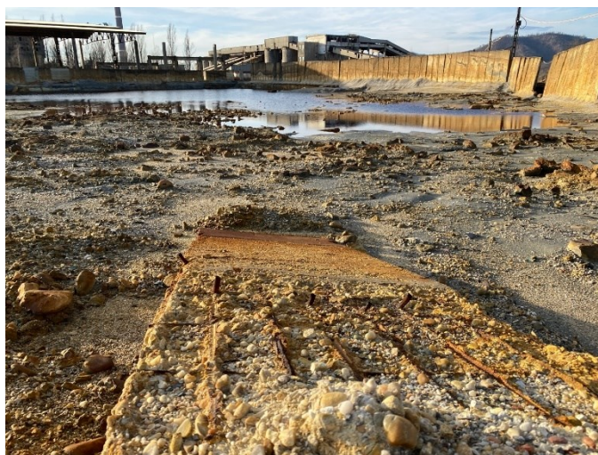
Figure 3 Framing the site in the natural landscape of Baia Mare and the presence of acidic waters and the impact on concrete
