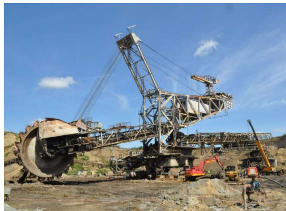
Fig. 1 The excavator with rotor type ERc 1400-30 / 7
