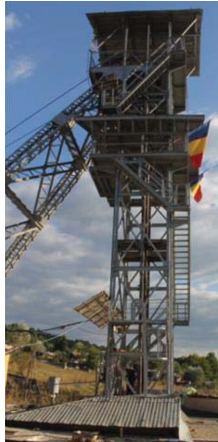
Fig. 8. The extraction installation tower at Unirea shaft
