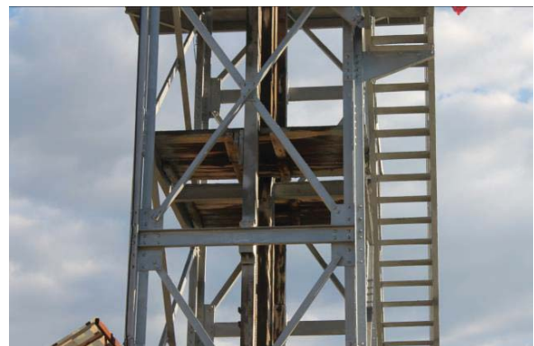
Fig. 12. Bridge for storage and oiling
