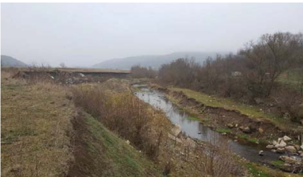
Fig. 1. Active erosion in the area of the assessed location
