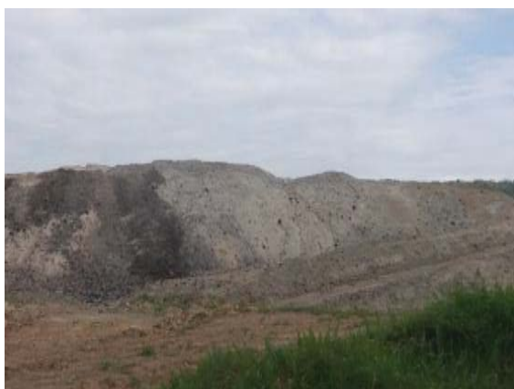
Fig. 2. Erosion processes on Panga inner dump
