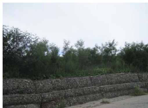
Fig. 5. Consolidation of the inner dump from Olteț with stone walls, reinstallation of the forest vegetation with modified structure
