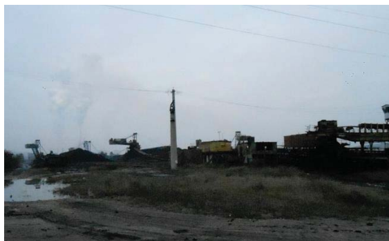
Fig. 2. Crushing coal deposit
