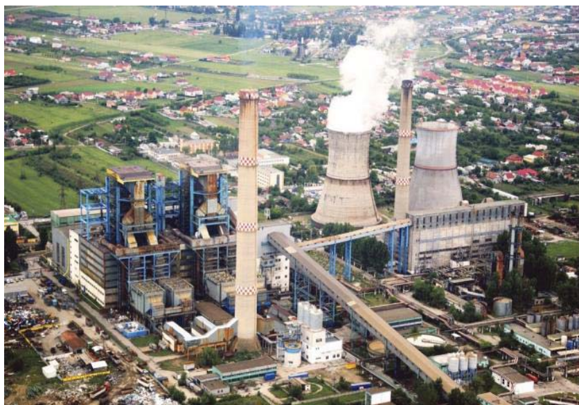
Fig. 1. Overview of the Rovinari thermal power plant
