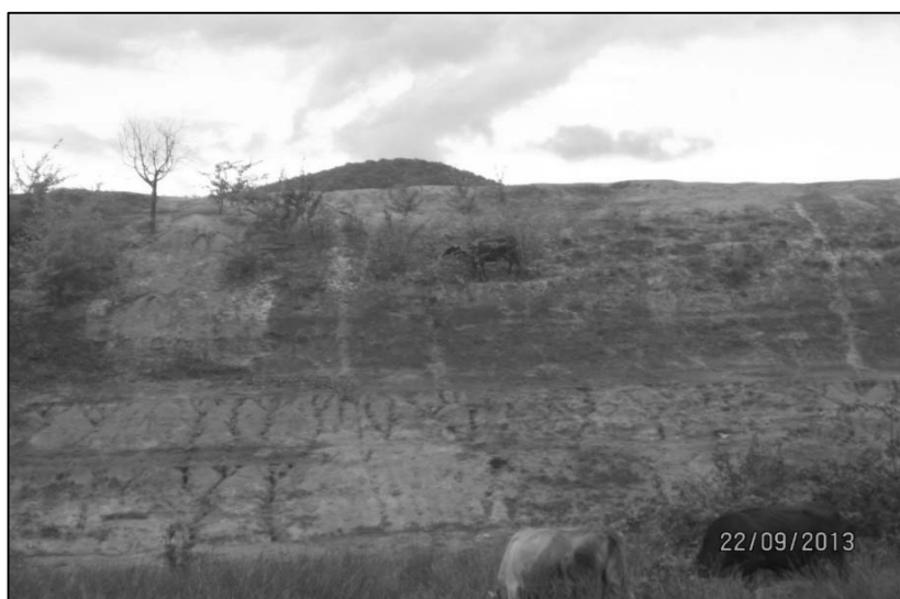
Fig. 10 The south slope of the Central tailing ponds (photo Irina Smical)
