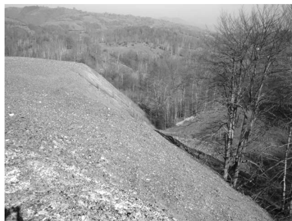
Fig. 5 Eastern and western slopes
