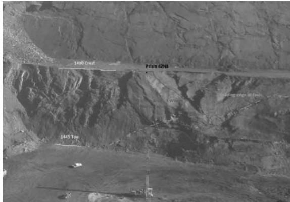
Fig.15. Pre-failure photograph of May 5, 2014 event showing location of Prism 42N
