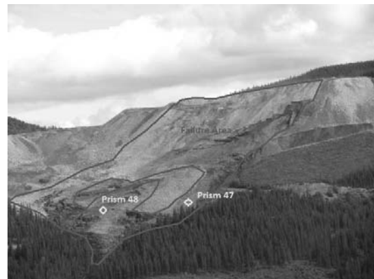
Fig.18. Post failure photograph, July 27, 2011, showing the location of monitoring prisms 47 and 48
