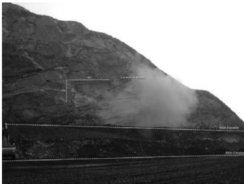
Fig.21. Analysis area post failure, July 16, 2012
