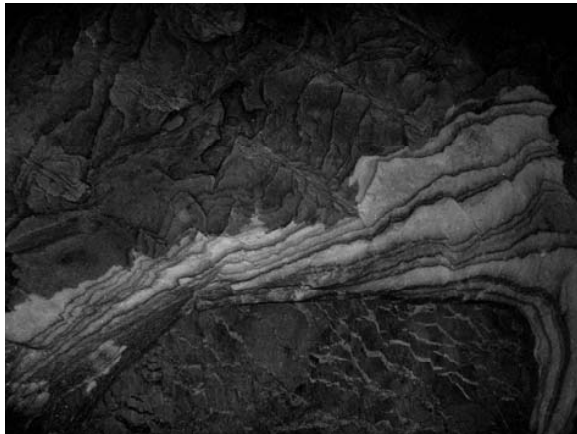
Figure 6. Ceiling fracturing phenomena
