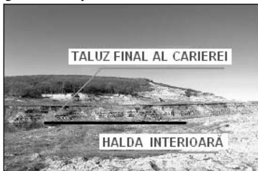
Figure 2. Sterile dumping in the inner dump of Ruget coal pit assisted in the final slope
