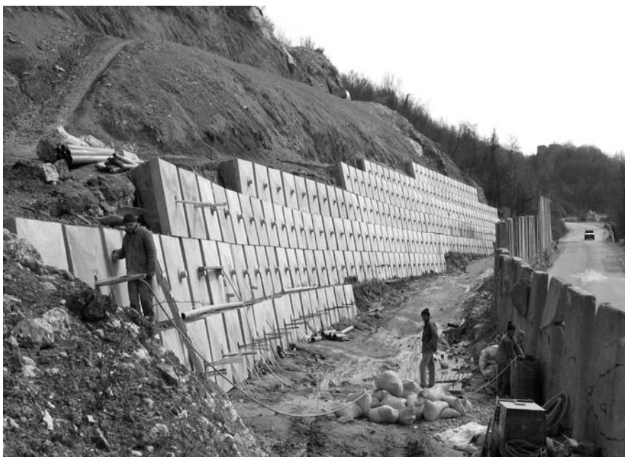
Fig.4. Mounting and fixing bolts
