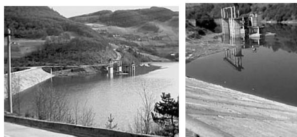
Fig. 1- The dam and the pond Mihoiești - overview
