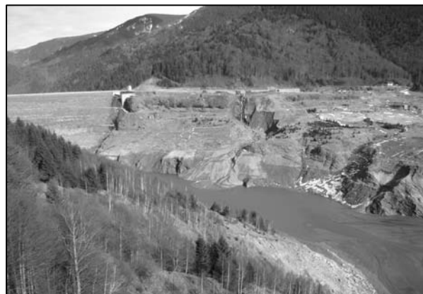
Fig.2 Location of the studied perimeter overview of the dam during emptying Gura Apelor
