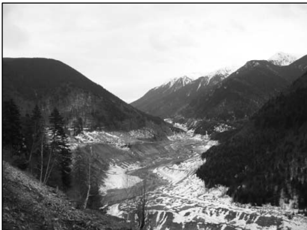
Fig. 4 Overview of the Ses River after emptying the dam Gura Apelor
