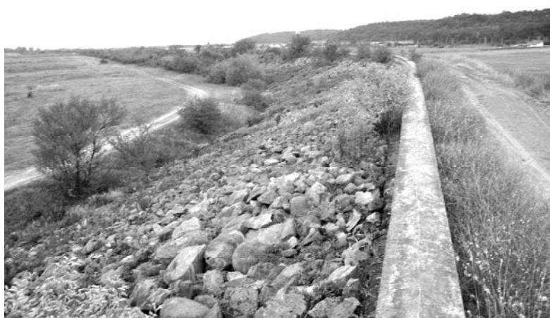
Figure 5 Protective measures with rocks filling-the retention dam of Jiu river in Rovinari area
