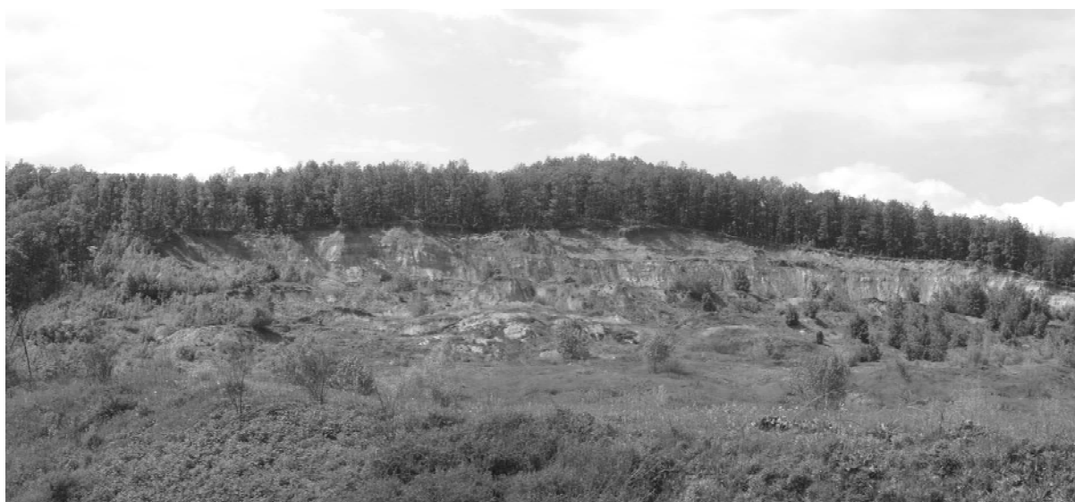
Fig.2; The micro-open mine Lupoița II, where frequently occurs landslides and rock fall
