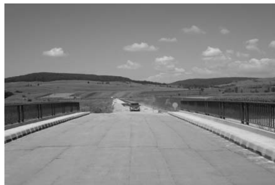
Fig.3. Sight on bridge
