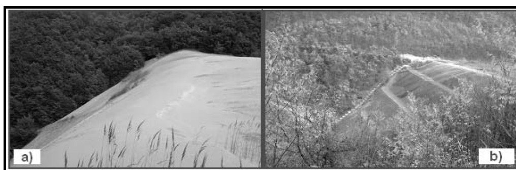
Fig. 6 The dam and crest of wave of Herepeia TMF E.M. Deva „Devamin”Subsidiary: a) before the work completion; b) after the finalisation of the environmental rehabilitation works
