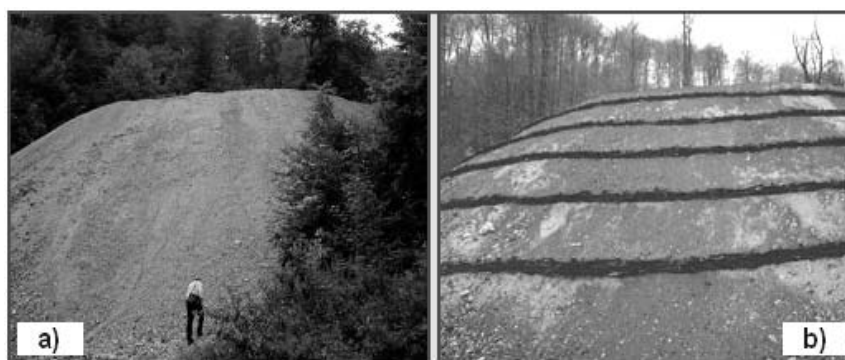
Fig. 4 Waste dump slope arrangement: a) before rehabilitation works; b) after rehabilitation works
