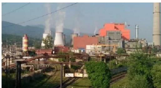
Fig. 1. Termocentrala Poroșeni ( https://www.economica.net/ )
