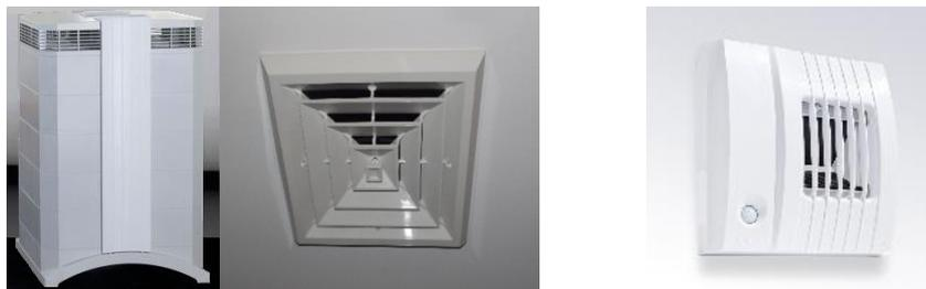
**Fig.2.** Ventilation system components of the hospital room: PAC (left), HVAC air intake port (center), HVAC air exhaust port (right)
