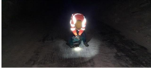
**Fig. 2.** Drilling the holes in the gallery floor
