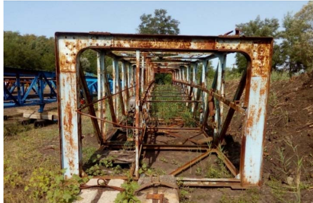
Fig. 1. Conveyor gangway truss bridge to be assessed
