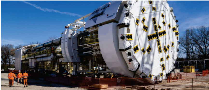
Fig. 1. TBM used for the modernization of the Apața – Cața railway section, Brașov county
