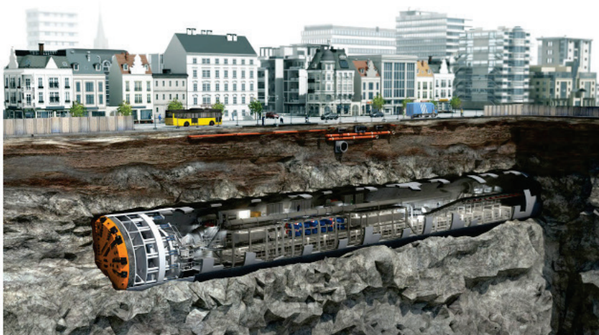
Fig. 2. Excavation mode using the TBM
