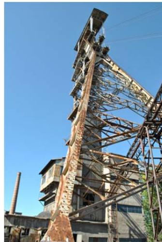
**Fig.3** The headframe of a mine winding machine
