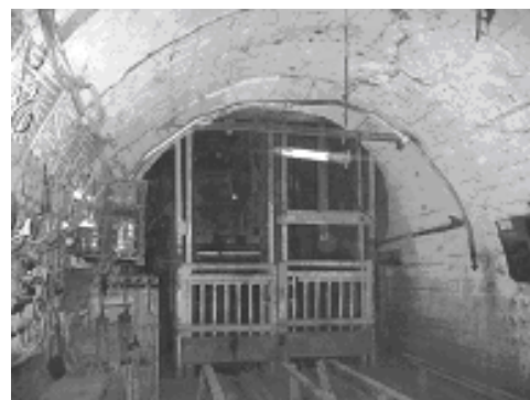
Fig. 1. Shaft ramp - 18 horizon (level - 15,744)
