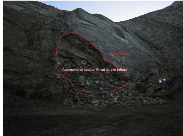
Figure 13. Post failure photograph of June 30, 2006 event, showing approximate original location of Prism 41
