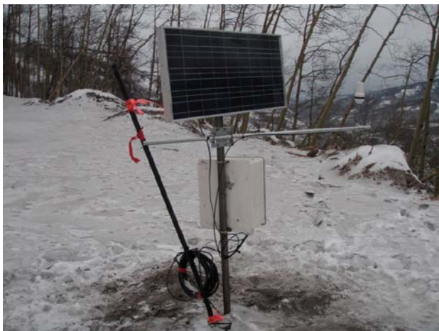
Figure 6. Remotely monitored vibrating wire piezometer
