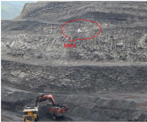
Figure 5. SSR-X radar monitoring a pit footwall from an access ramp
