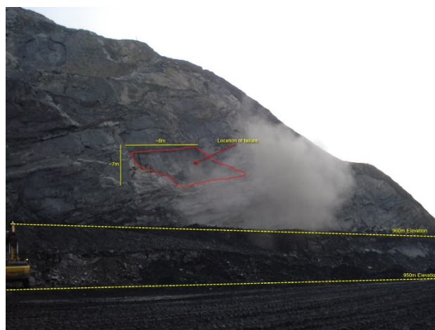
Figure 21. Analysis area post failure, July 16, 2012
