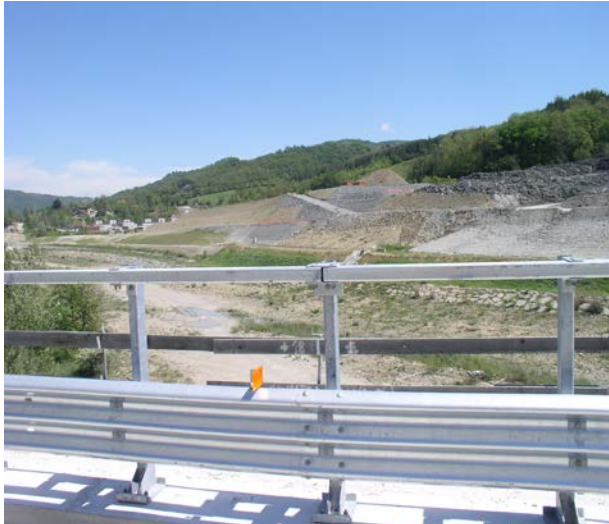
Figure 2. Embankments and ramps in road construction project in central Italy (Oggeri, 2012)
