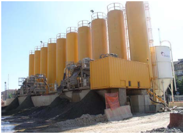
Figure 4. Compact slurry treatment plant (dewatering, fines separation and partial bentonite recycle) installed for Turin Railway "Passante" works (Oggeri, 2009).
