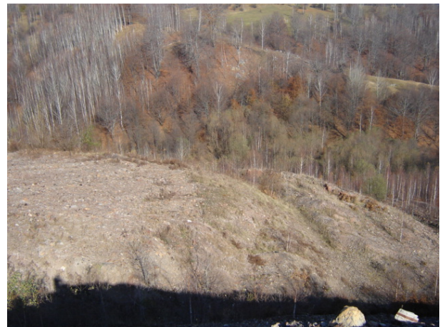
Photo 5 Sliding area on the eastern slope
