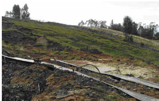
Photo 6 Discharge phenomena and slope ruptures
