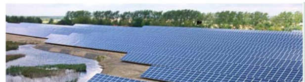
Fig.14. PV system in Espenhain Germany
