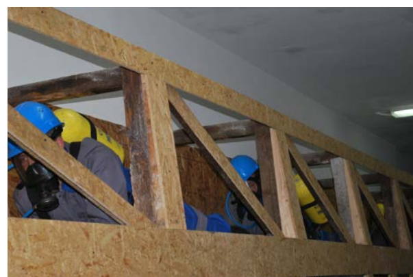
Fig. 12 - Moving in confined spaces
